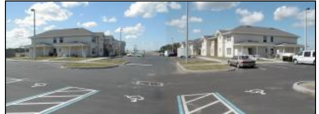
Wycliffe Apartments – Our Temporary Home
