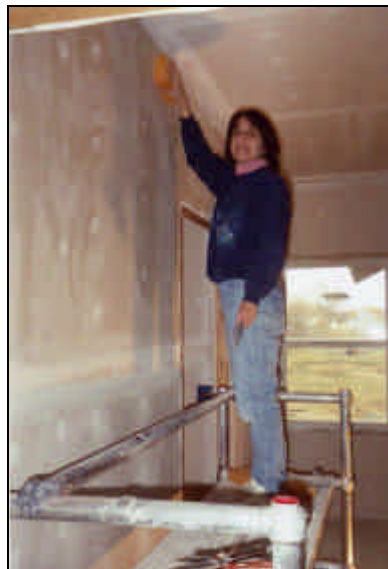
Barb Busy With Drywall Work
