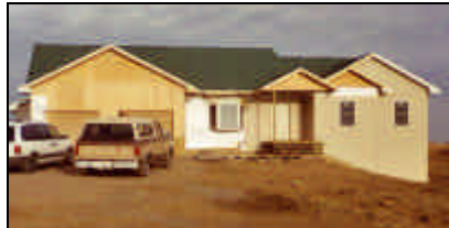
Eastling's New House
